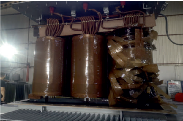
On-site Transformer Controls and Burnt Transformer Repair
