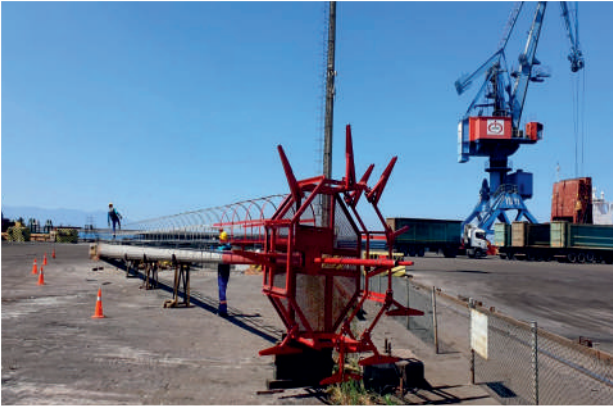
İsde mir 17 Pole Perimeter Lighting
