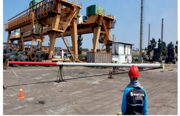
İsde mir 17 Pole Perimeter Lighting
