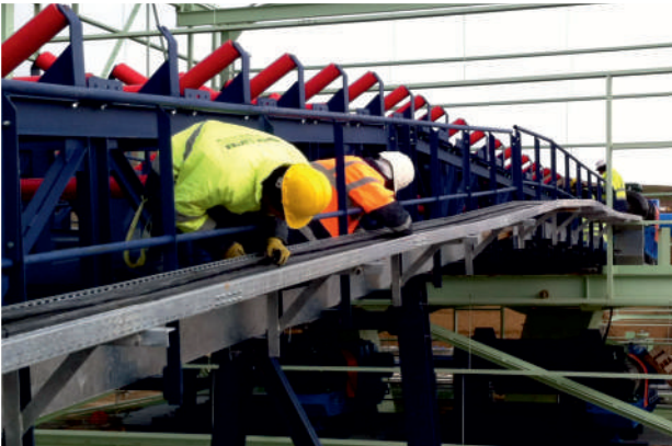
Cable Pulling Process
