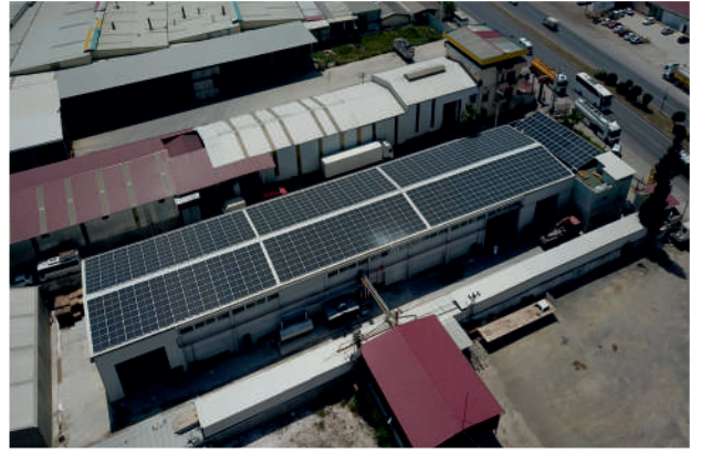
Serven SPP / 295,2kWp
