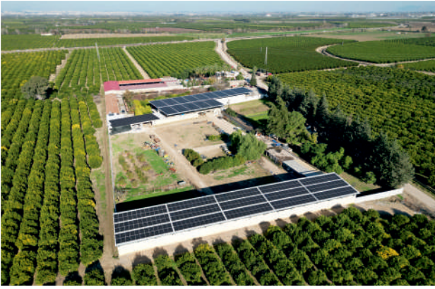
Ramazanoğlu SPP / 597,87kWp
