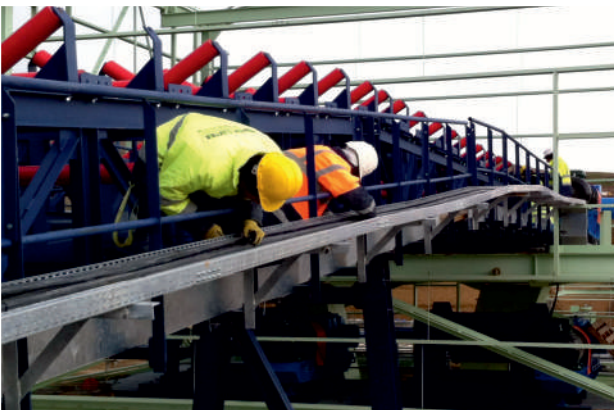
Cable Pulling Process
