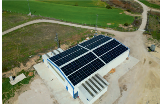
Tayftar Agriculture SPP / 174,4kWp
