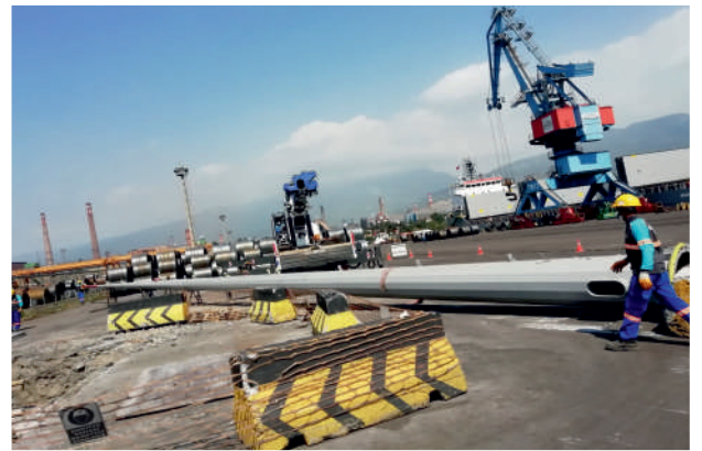
İsdemir 17 Pole Perimeter Lighting
