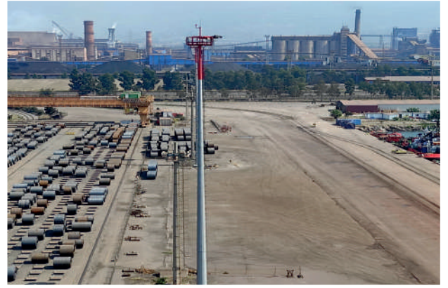
İsdemir 17 Pole Perimeter Lighting
