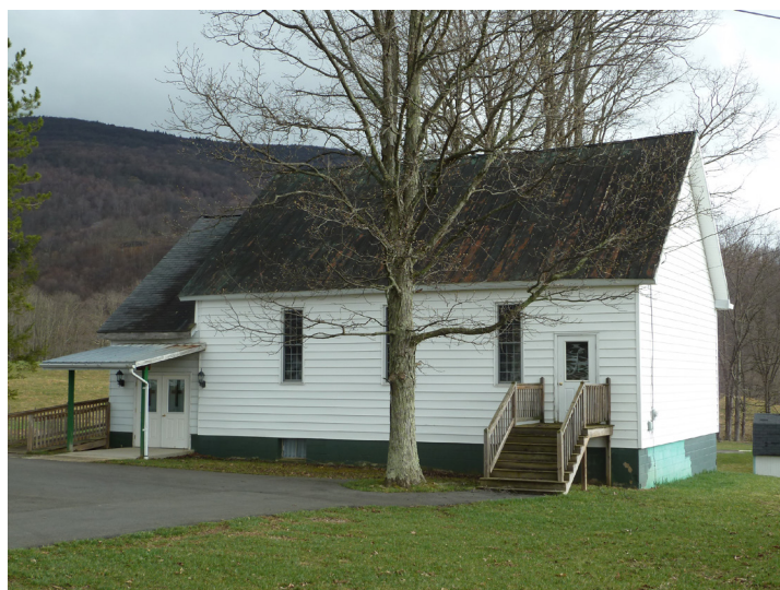
Former Lanesville Mennonite Church, West Virginia,
