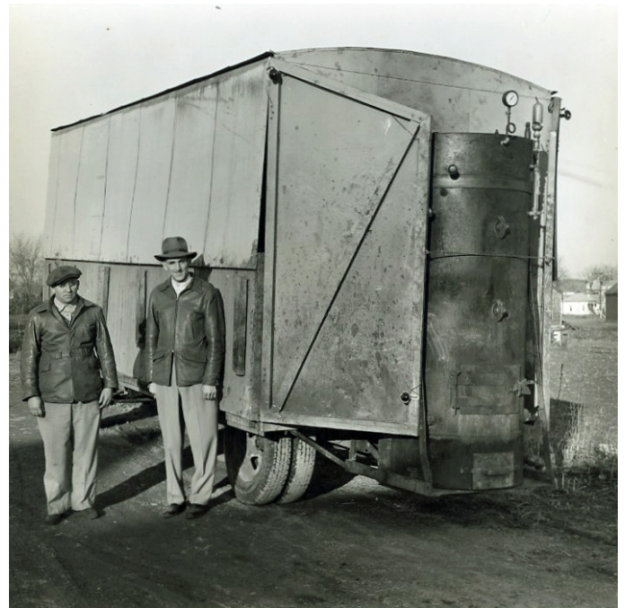
Lewis Martin (right) and an unidentified man stand beside the Virginia Portable Canner in the 1940s, with the chimney removed for travel.
