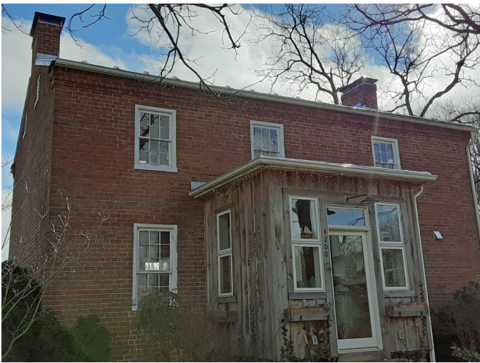
The historic Wenger house, Rockingham County, Va, near Greenmount Church of the Brethren and the Brenneman-Turner Mill. The house dates to 1857. This west porch was added in 2015. Occupants of the house are the Peter and Bethany Versluis Fairfield family.
