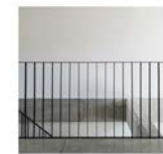
FE06 POWDERCOATED STEEL BALUSTRADE
