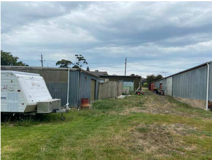
11 View of site at 30 Geelong Rd
