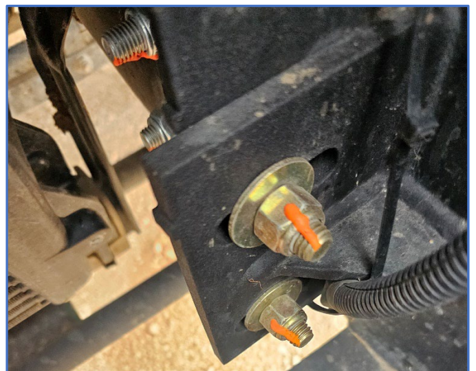
Top Photo – Rear stabilizer link with missing nut and damaged threads.
