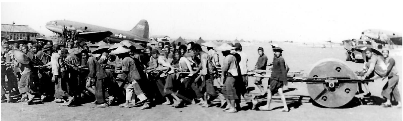
An iconic Hump scene: Chinese coolies rolling the strip at the Kwangan airfield. C-46s in the background. Frank D. Martin 1944
