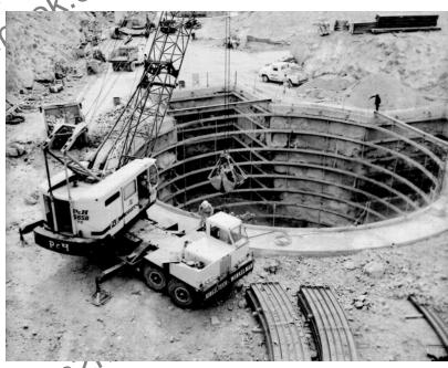
and structure of the silo wall. At the bottom of the silo, a  $\frac{1}{4}$ -inch (6 mm) thick steel plate floor was installed for electromagnetic pulse (EMP) shielding. Extending up from this floor, steel plates were attached to the ring beams to form a metal cylinder that extended all the way to the surface.<sup>12</sup>
