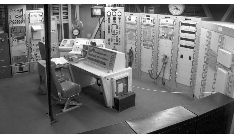
▲ The launch control center (LCC). The control complex facilities console (LCCFC) is at center.
