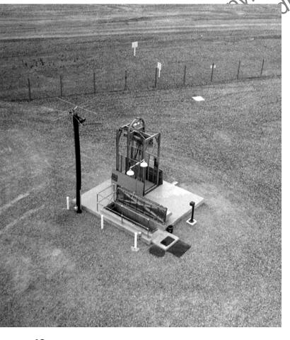
and phone; the entrapment area, telephone and closed-circuit TV camera; the stairway; the elevator; and a blast door with its associated phone. Also located within the access portal was an exhaust fan with its vent hood on the "roof" of the portal and a sump pump located at the bottom of the elevator shaft.
