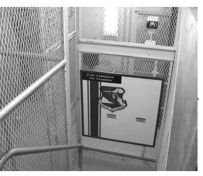
▲ Looking into the entrapment area from the outer portal door. Note TV camera. the *entrapment area*, which confined those entering until their authorization to enter could be confirmed. The entrapment area consisted of two electrically locked doors, one at each end of a short stairway. When the outer door closed, those inside were trapped between it and the inner door. Both doors had to be buzzed open with a button in the LCC, but both doors could not be unlocked at the same time
