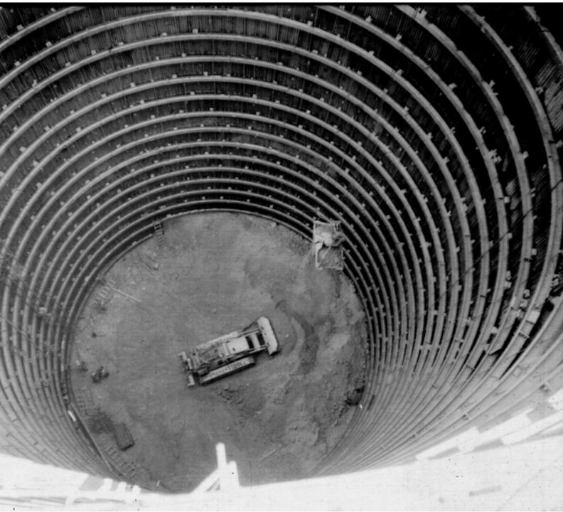
▲ Ring beams formed the outline of the silo wall, and supported the silo's exterior steel shell. Note bulldozer at bottom, and lift bucket.
