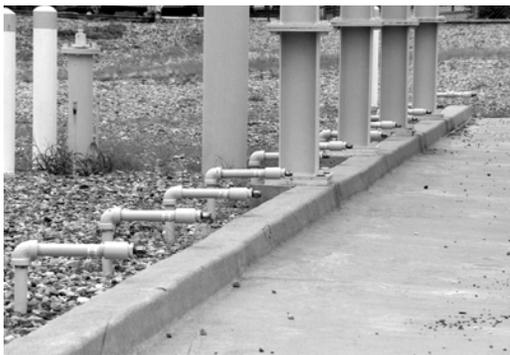
*hardstands.* These served as parking areas for the tank trucks and holding trailers used to load and unload missile propellant. Fuel was loaded from the east hardstand and oxidizer from the north. The most obvious difference between the two was the fuel hardstand's water spray nozzles. These nozzles were used for fire suppression and to wash down equipment
