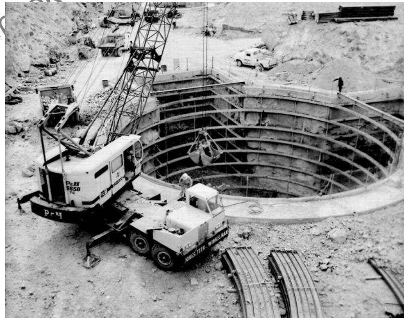
and structure of the silo wall. At the bottom of the silo, a ¼-inch (6 mm) thick steel plate floor was installed for electromagnetic pulse (EMP) shielding. Extending up from this floor, steel plates were attached to the ring beams to form a metal cylinder that extended all the way to the surface.<sup>12</sup>
