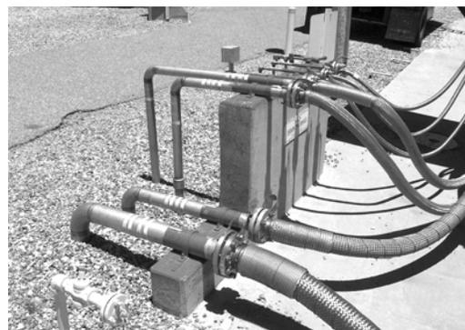
◀ Propellant was loaded into the missile by gravity via stainless steel piping. The larger of the two pipes in the foreground is for stage one, the smaller one for stage two.
