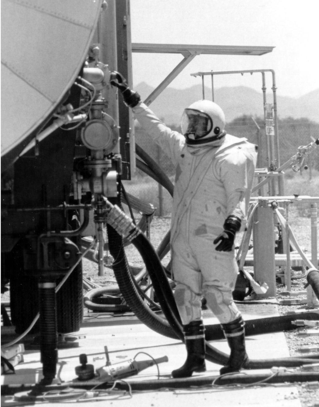
◀ The rocket fuel handler's clothing outfit, or RFHCO, worn to protect against the highly toxic vapors of the propellant. The suits were not air-conditioned.
