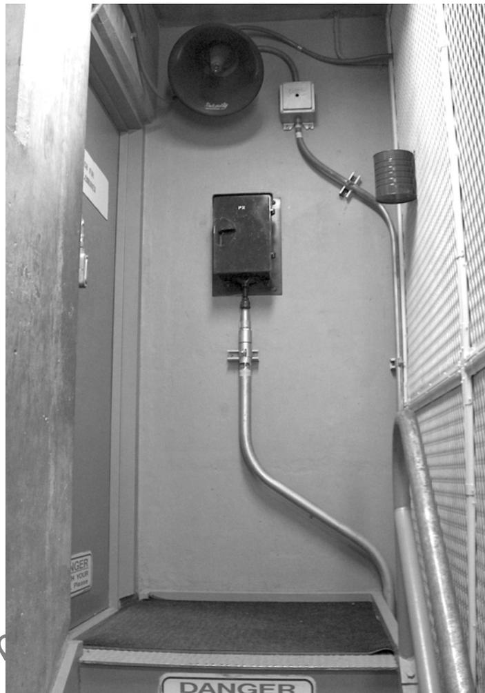
▲ Looking up from inner door. Note telephone and VSS speaker at top of stairway, and burn can at right.
