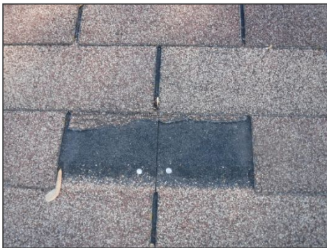
Roof Covering Missing Shingles (Front Side)
