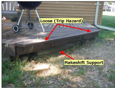
Deck not property supported / loose edge board (trip hazard)
