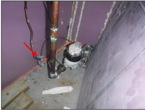
Bonding clamp not secured to water pipe
