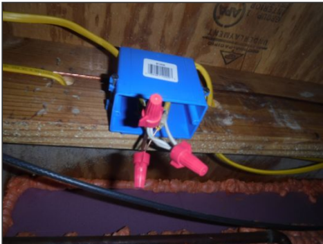
Junction box missing cover
