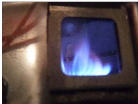
Example Of Water Heater Burner In Operation
