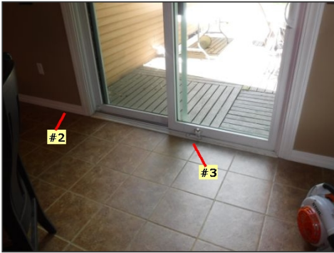
Approximate Interior Location #2 & #3 (Above Stained Sub-floor/Rim Joist)
