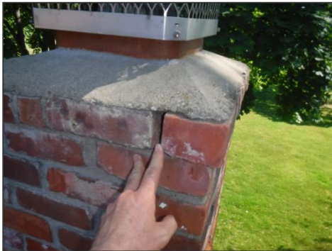
Delayed Maintenance, retuck mortar joint.
