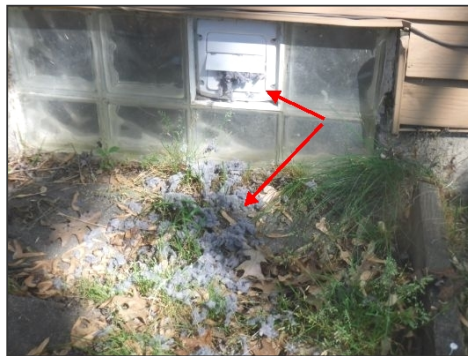
Dryer vent obstructed with lint (safety Hazard)
