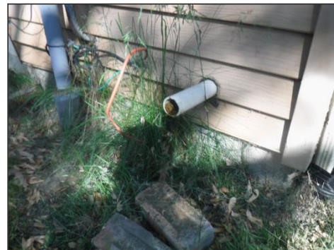
Example Of Sump Pump Discharge Pipe To Close To Foundation
