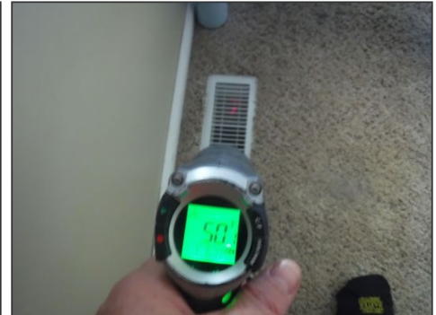
Cooling air temperature during operation (50 degrees)
