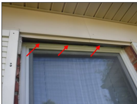
Delayed Maintenance, front windows, missing caulking
