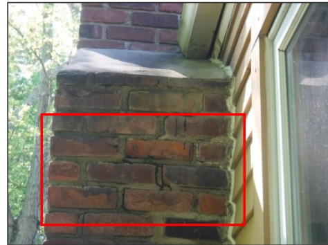
Delayed Maintenance, retuck mortar joint.
