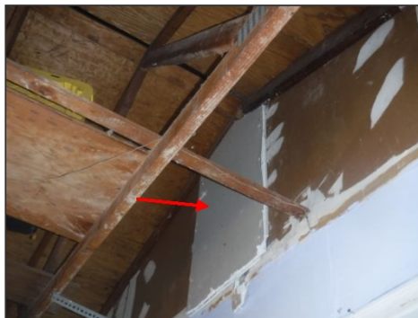
Garage, attic secured by drywall panel (I did not access the attic)
