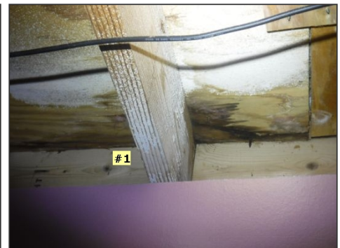
Location #1, Stained sub-floor (Below bedroom)
