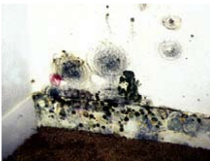
mold on a wall
