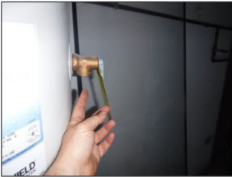
Missing discharge tube
