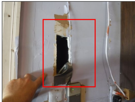
Garage, breach in firewall
