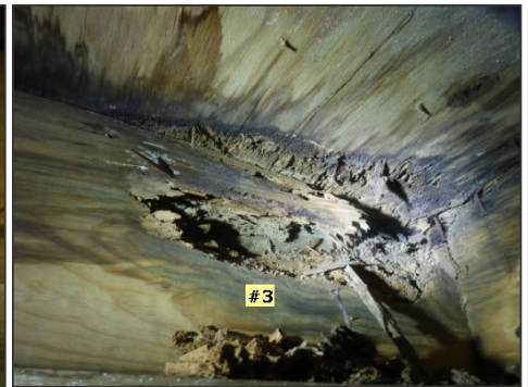
Location #3 (Structural Damage), damage sub-floor/Rim Joist (below glass door wall)
