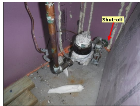
Example Of Water Service Meter And Shut Off Valve
