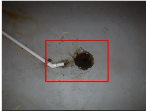
Discharge tube need extension to the floor drain
