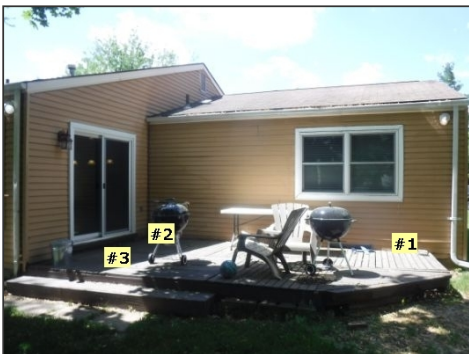
Approximate Exterior Location #1, #2, & #3 (of Stained Sub-floor/Rim Joist)
