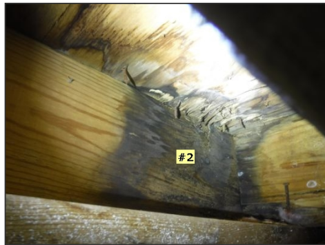
Location #2 (Structural Damage), Elevated moisture, damage sub-floor/Rim Joist (Left side of door wall)
