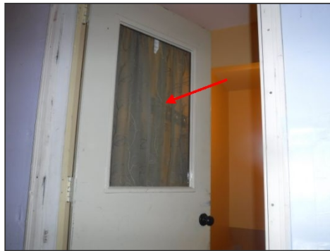
Garage occupant not fire rated (Glass Panel)
