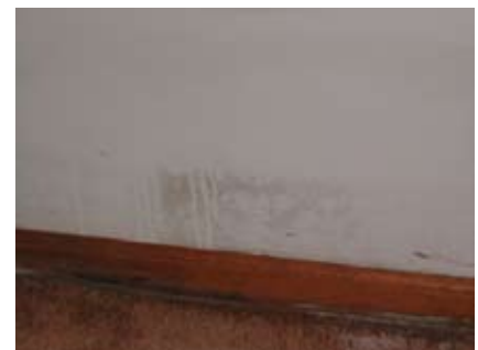
mold on a wall and carpet
