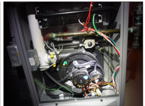
Example of Heating System With Service Panel Removed
