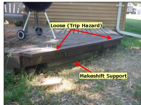
Deck not property supported / loose edge board (trip hazard)
