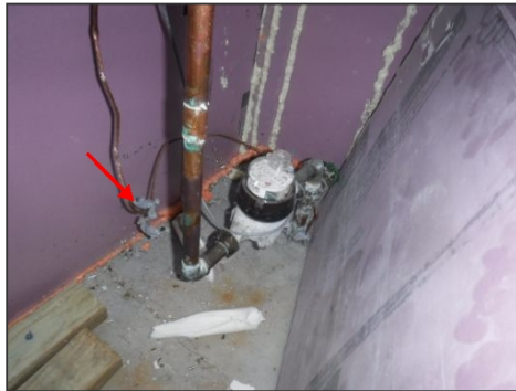
Bonding clamp not secured to water pipe
