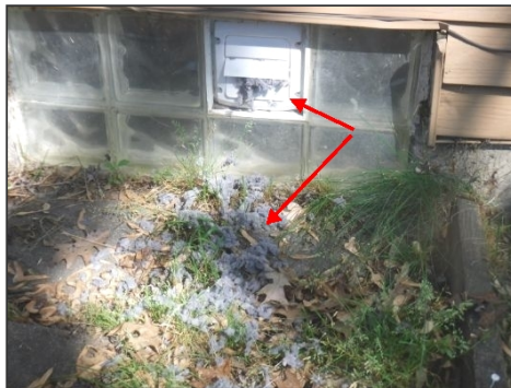
Dryer vent obstructed with lint (safety Hazard)
