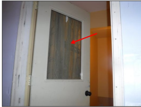
Garage occupant not fire rated (Glass Panel)
