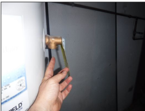
Missing discharge tube
