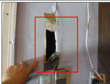
Garage, breach in firewall
