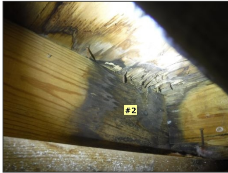
Location #2 (Structural Damage), Elevated moisture, damage sub-floor/Rim Joist (Left side of door wall)
