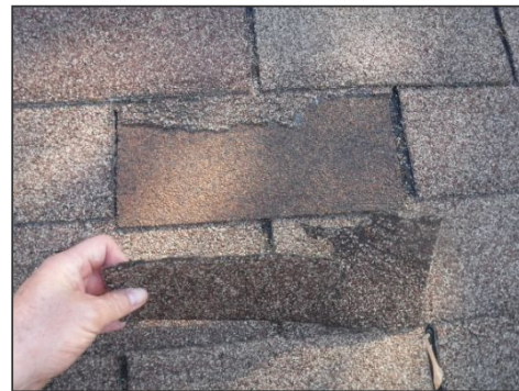
Roof Covering Missing Shingles (Front Side)
