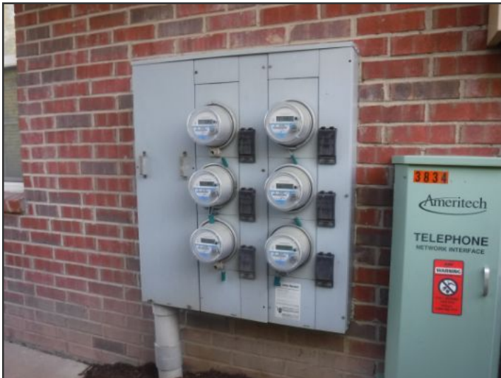
Example Of Service Meters
