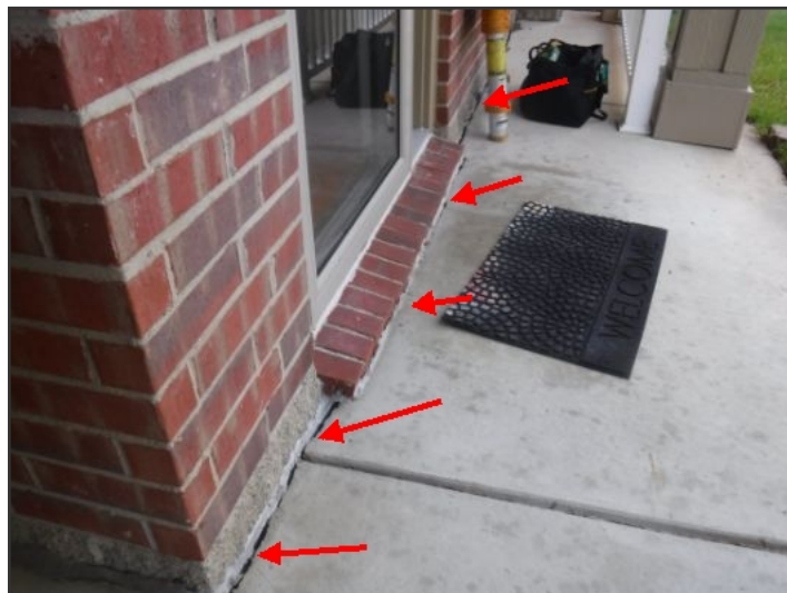
Caulking needed (Front Entry)
