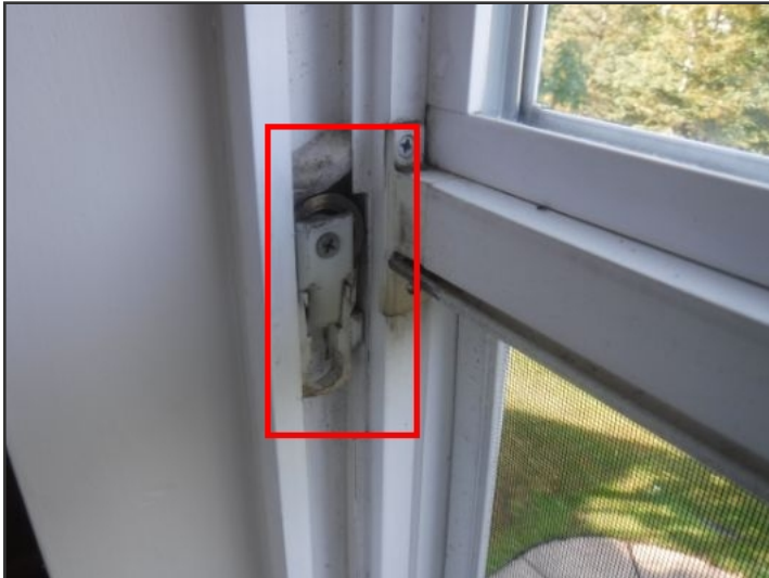
Broken window left side sash (Master Bedroom, left window)
