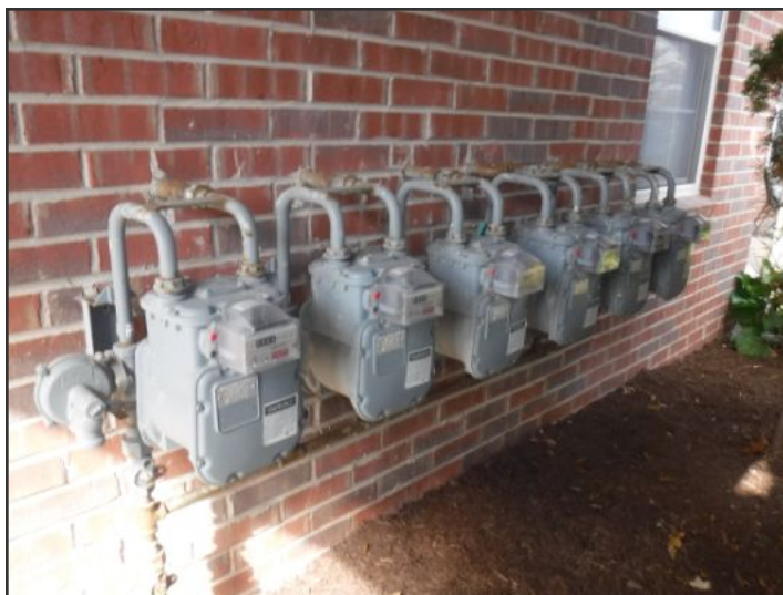
Example Of Gas Service Meters And Shut Off Valves
