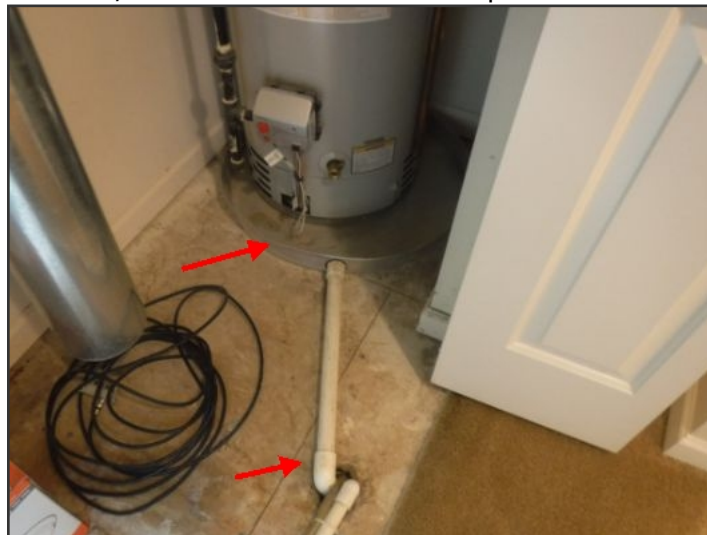
Drip pan and drain to floor drain
