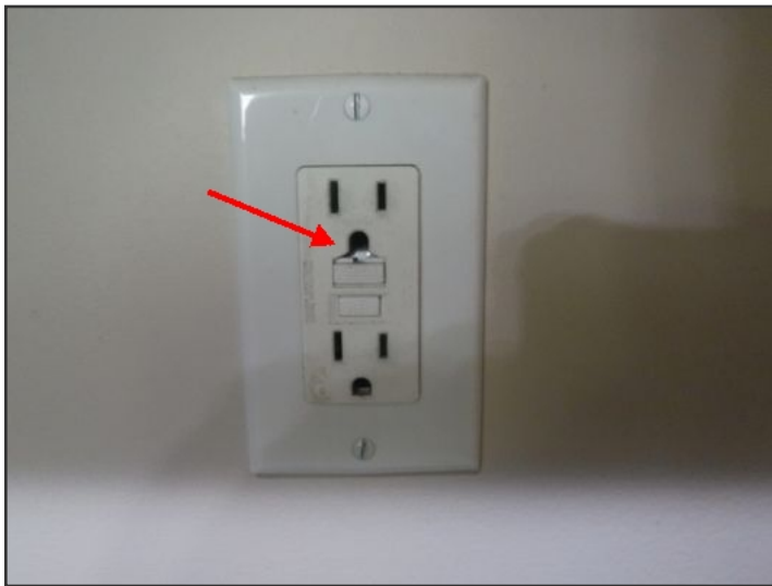
Kitchen, damage GFCI protected outlet (right side of refrigerator)
