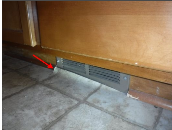
Upstairs common bathroom floor (linoleum lifted)
