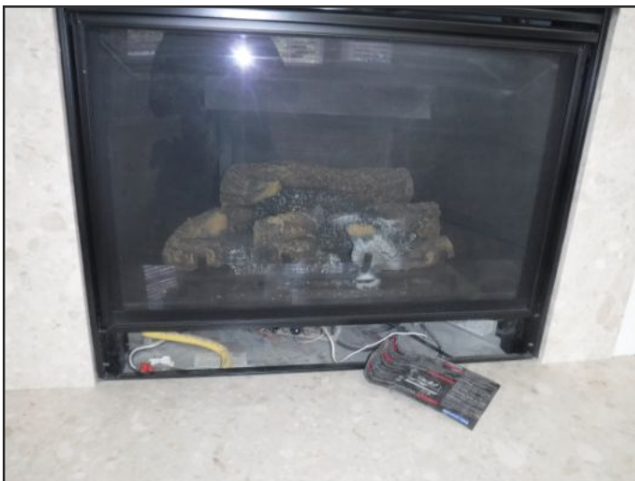
Example gas fireplace with lower gas control/ shut-off valve
