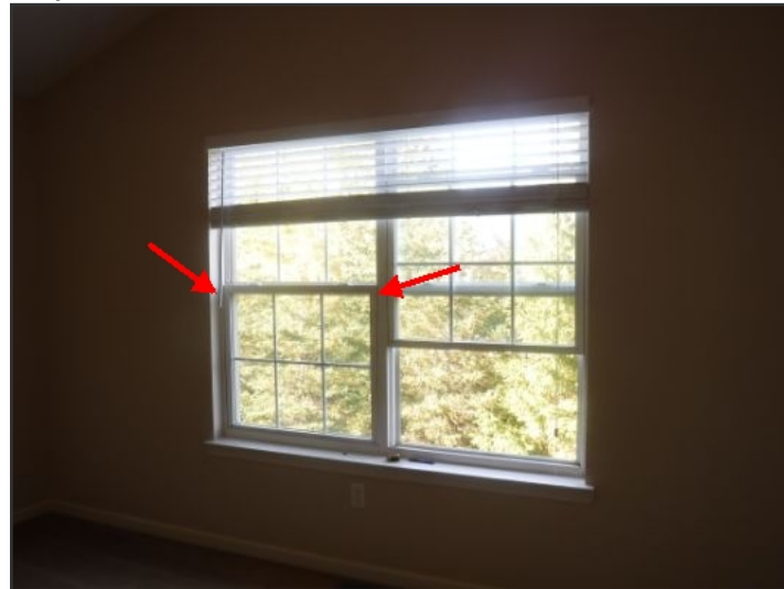
Broken sash (Master Bedroom, left window)
