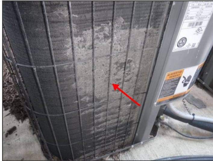
Example Of A/C Unit dirty fins
