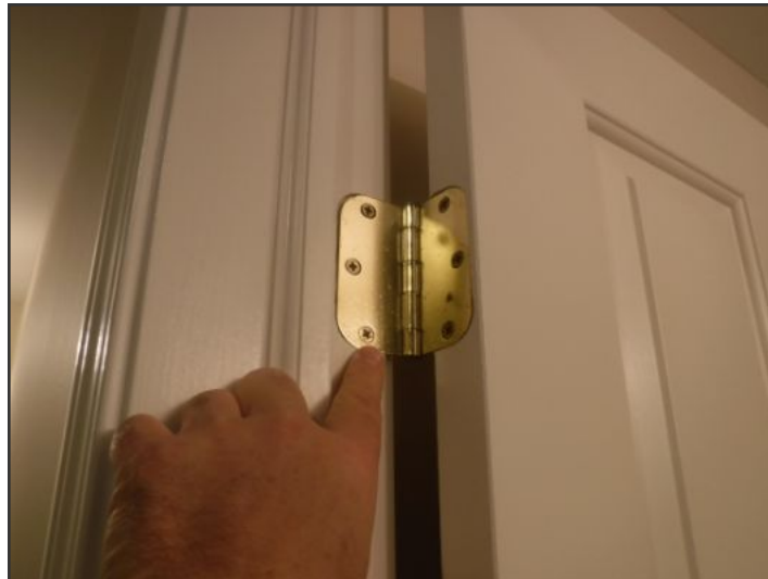
Upstairs common bathroom loose upper hinge
