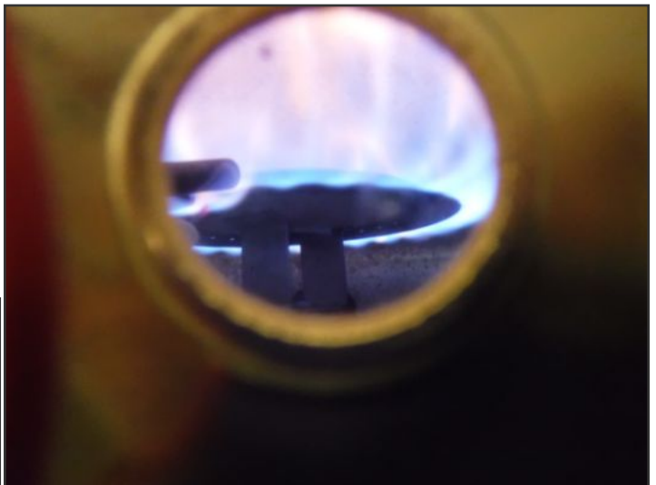
Example Of Water Heater Burner In Operation
