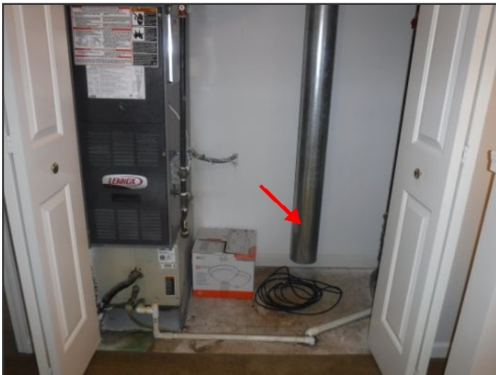
Example of Heating System Make Up Air Duct (Do Not Block)
