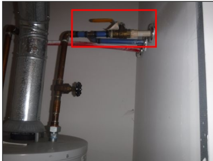
Example Of main shut off valve
