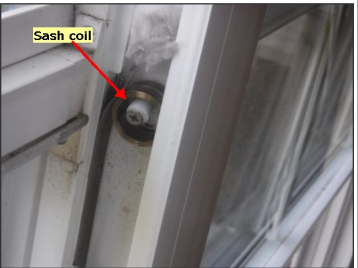
Broken window right side sash coil (Master Bedroom, left window)
