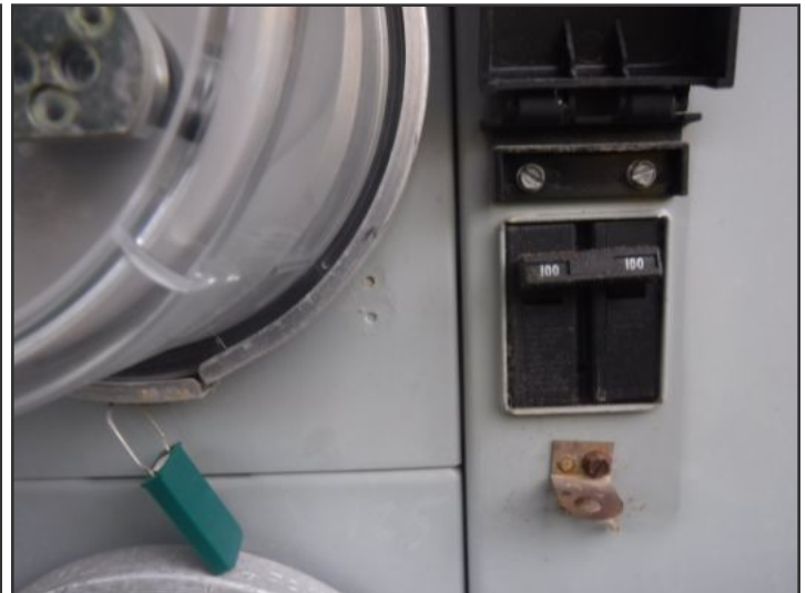
Main Breaker at meter (100 amp)
