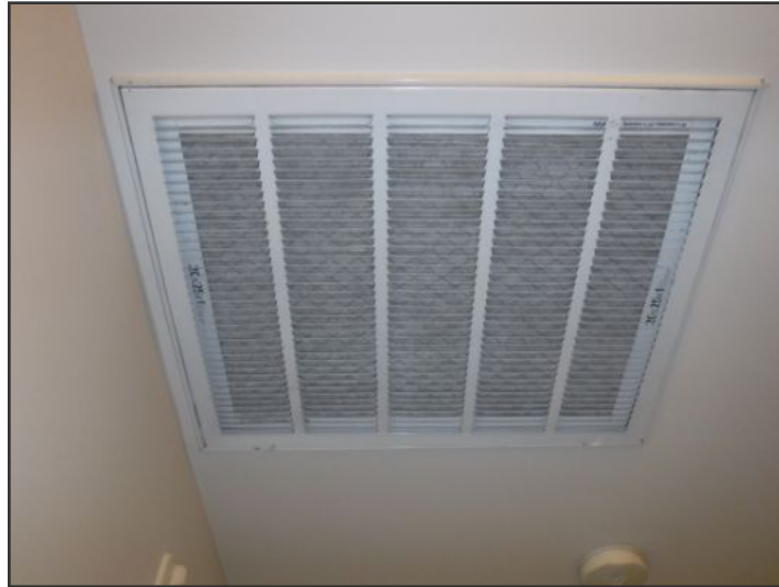
Ceiling access to air filter (upstairs hallway)
