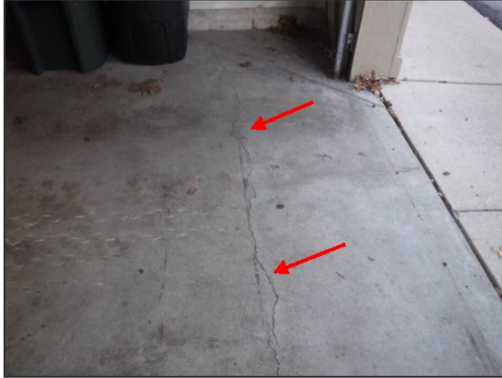
Example Of Garage Floor stress cracks (No Trip Hazard)
