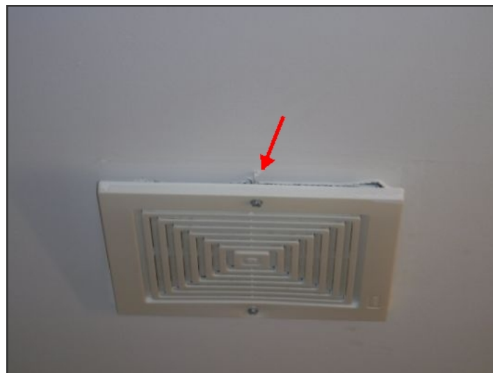
Upstairs common bathroom loose ceiling fan grill
