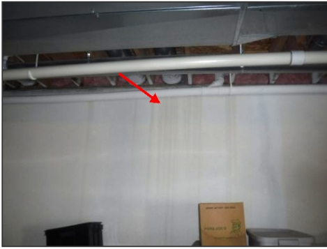
Dried moisture stains
