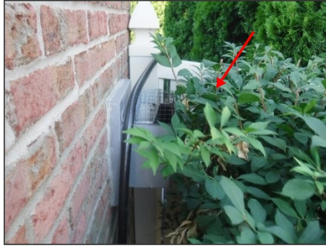
Trim away bushes from fireplace exhaust vent (Right Side)
