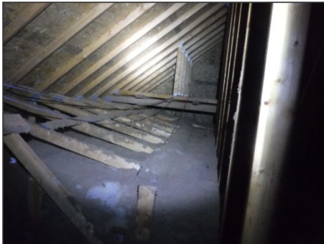
Example Of Attic Insulation
