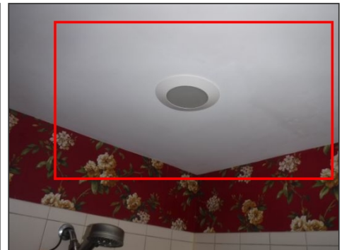
Master bathroom show ceiling (Patched area)
