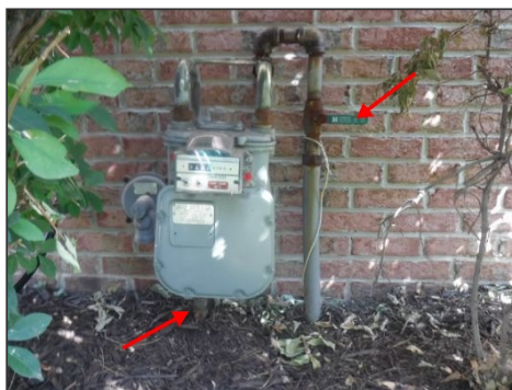
Example Of Gas Service Meter And Shut Off Valve
