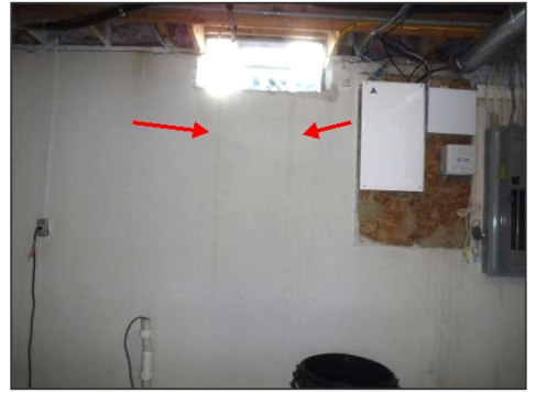
Dried moisture stains
