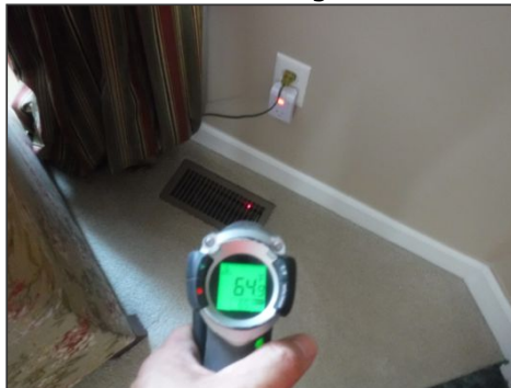
Heating air temperature during operation
