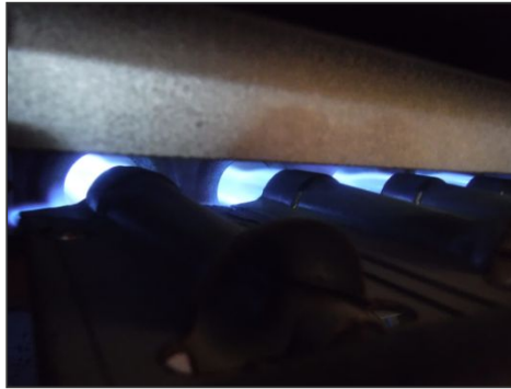
Example Of Furnace Burner In Operation
