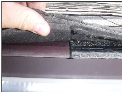
Example Of Roof Covering (Single Layer)
