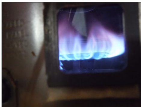
Example Of Water Heater Burner In Operation
