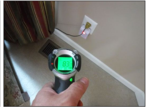
Heating air temperature during operation
