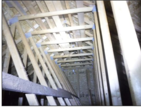
Example Of Roof Structure Within Attic
