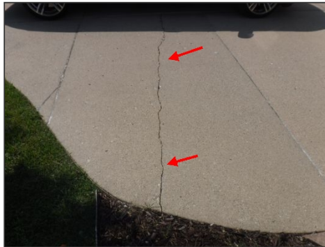
Example Of Driveway Crack, No Trip Hazard
