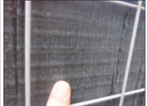
Fins damaged (Close-up)
