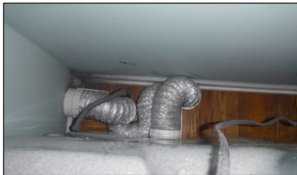
Example Of Foil Dryer Duct
