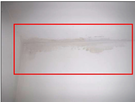
Den Ceiling Stain (Dried stain)
