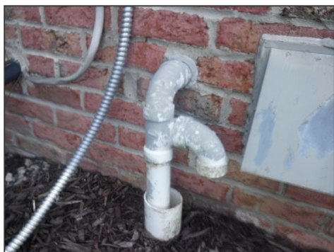
Example Of Sump Pump Exterior Discharge
