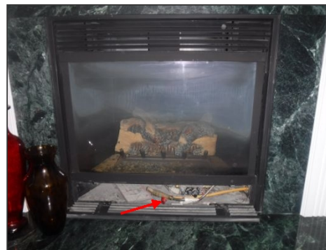
Example of gas log set controls and gas shut-off valve for future reference
