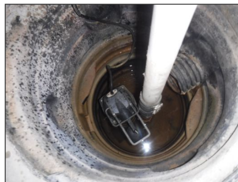
Example Of Sump Pump And Basin
