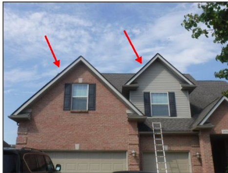
No access to roof cavities
