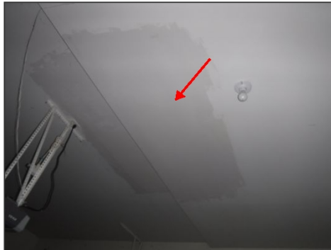
Patched/repair ceiling area
