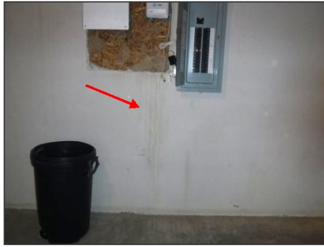
Dried moisture stains
