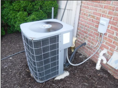
Example Of A/C Unit
