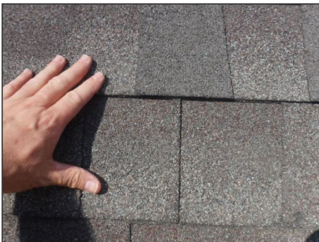
Example Of Roof Covering
