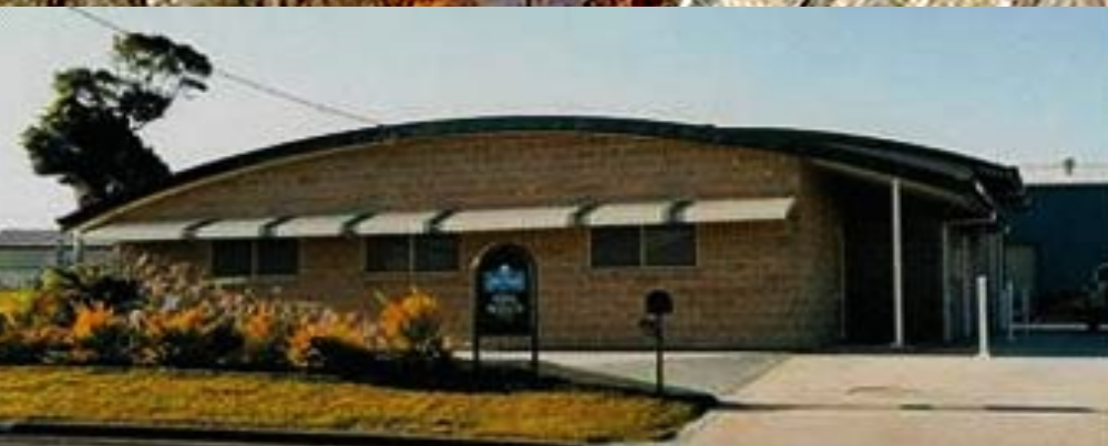
Image of the GMP certified manufacturing facility in northern NSW.
