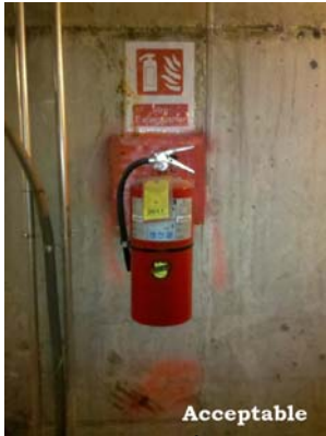
Fire extinguisher in a construction site.
