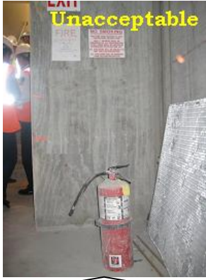
Improper floor placement of Fire Extinguisher.
