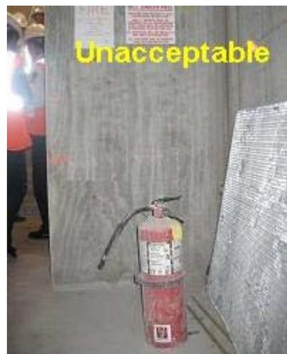
The bottom of the extinguisher must be at least 4 in above the floor.
