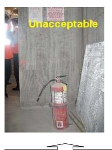
The bottom of the extinguisher must be at least 4 in above the floor.
