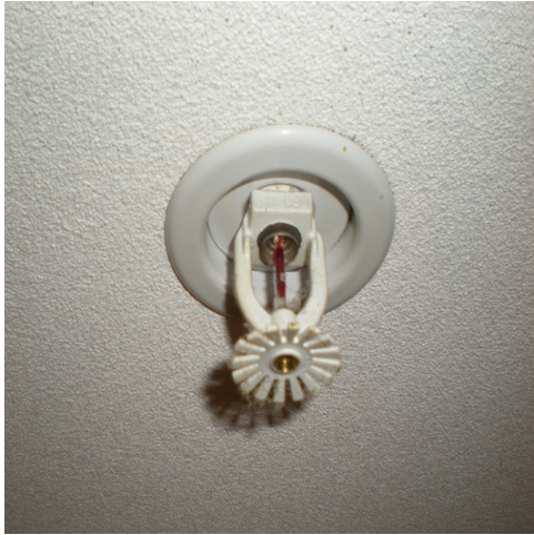
Factory applied finish sprinkler head
