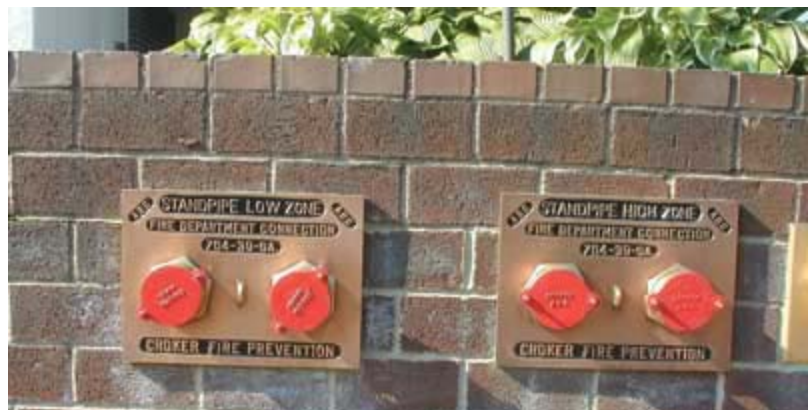
(The left Fire Department Connection in the photo is to cover the lower zone and the right Fire Department Connection is to cover the higher zone.)
