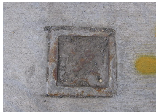
Gas shut-off valve in sidewalk
