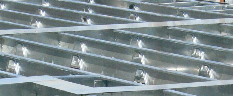
You can't always predict extreme weather or other construction-halting incidents. But you can create buildings that are durable and safe, even in the event of a disaster. The durability and resilience of cold-formed steel framing makes it an ideal material to stand up to cold-weather, high winds, flooding, and fire — during construction and throughout the life of the building.
