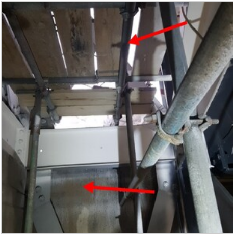
OUTSTANDING WORKS COMPLETE AFTER SCAFFOLD REMOVED
