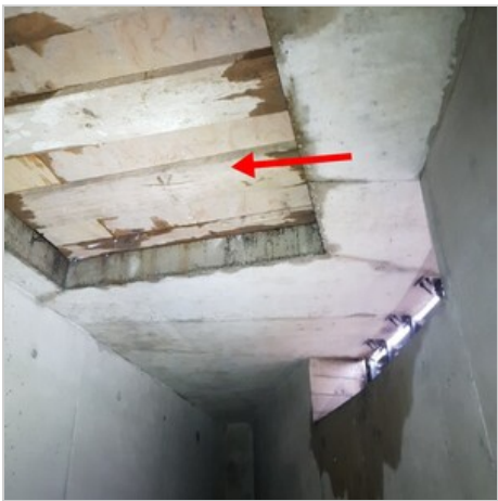
MISSING HATCH/PANEL
