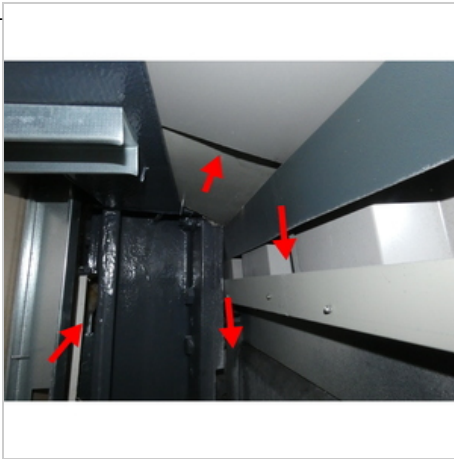
DAYLIGHT BETWEEN STEEL AND FLASHING'S
