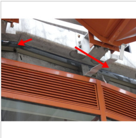
EXTERNAL VIEW - ZEFYR REMOVE DRIPPING FLASHINGS AND GUTTERS
