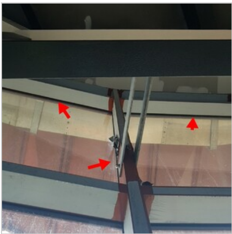
WATER DRIP THROUGH THE TRANSOM PLATES AND GASKET
