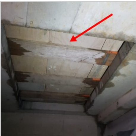
MISSING HATCH/PANEL
