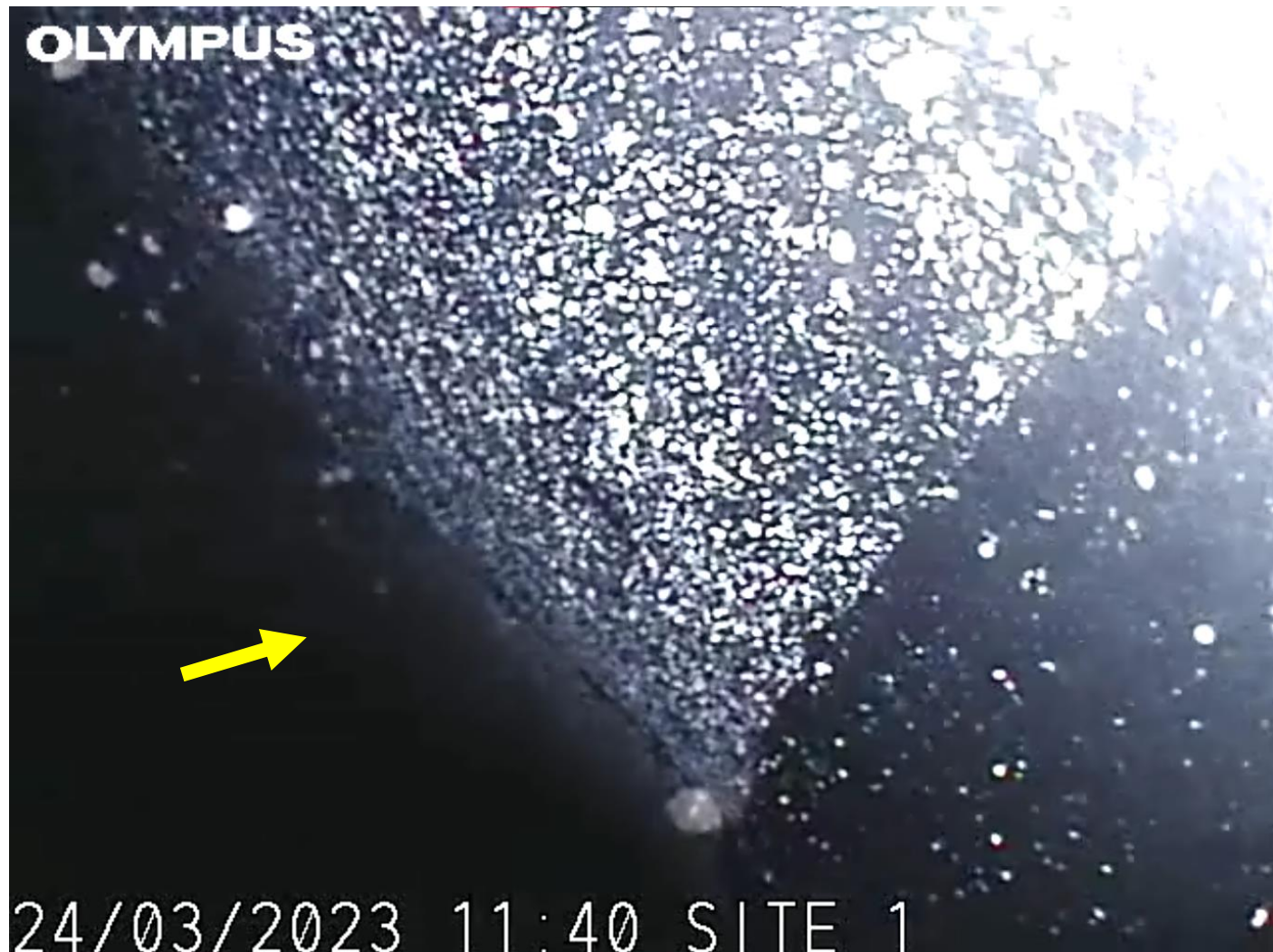
L Felt/membrane visible
