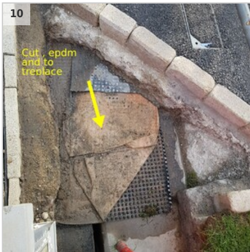
Cavity not complete. To be weatherproofed
