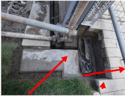
Missing Weatherproofing
