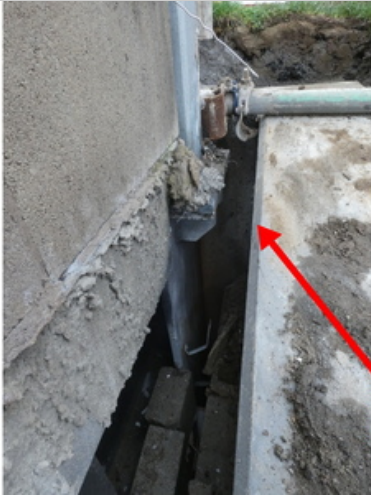
Cavity not complete. To be weatherproofed
