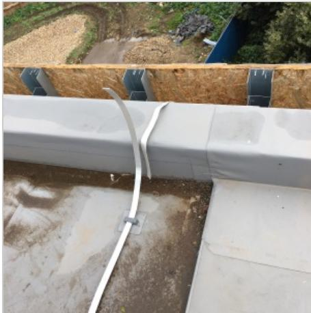
● **#277 - Panel Insulation exposed on weather condition , to be protect and not complete. Membrane and Coping to install.**
