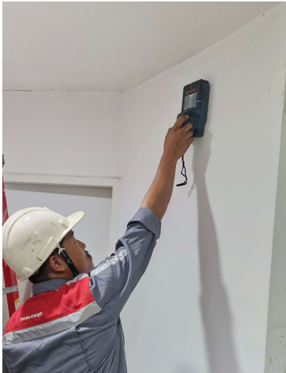
Wall scan before drilling
