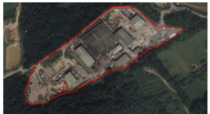
Figure 7: Aerial photo of the Allocated Site – Inset 8
