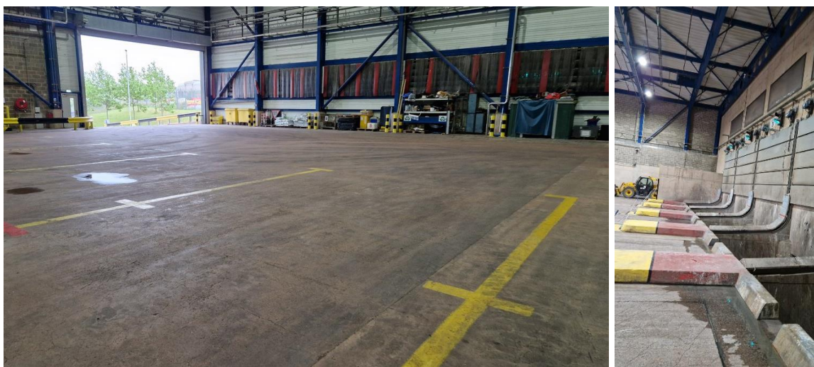
Graphic 2-1: MVV’s Devonport tipping hall including tipping bunker apertures (right)
