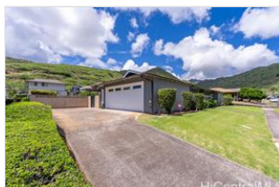
Slightly sloped driveway leads to enclosed 2-car garage with lots of storage and added privacy.
