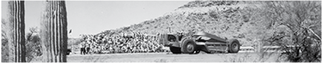
International Harvester 27-75 earthmover being demonstrated in front of a grandstand at International Harvester's Phoenix Proving Ground in 1953 (Credit: Wisconsin Historical Society. Image ID 39941)
