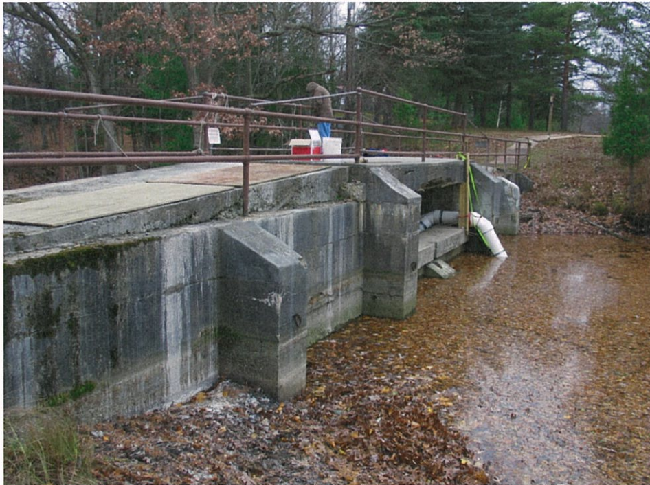
Upstream Face – Looking south-westerly
