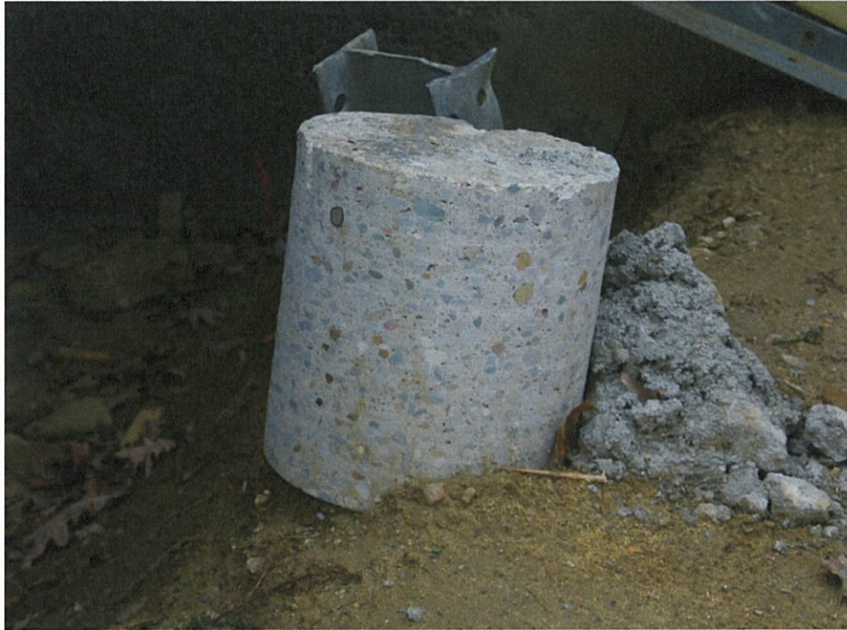
Deck Core – Typical of 8 cores taken
