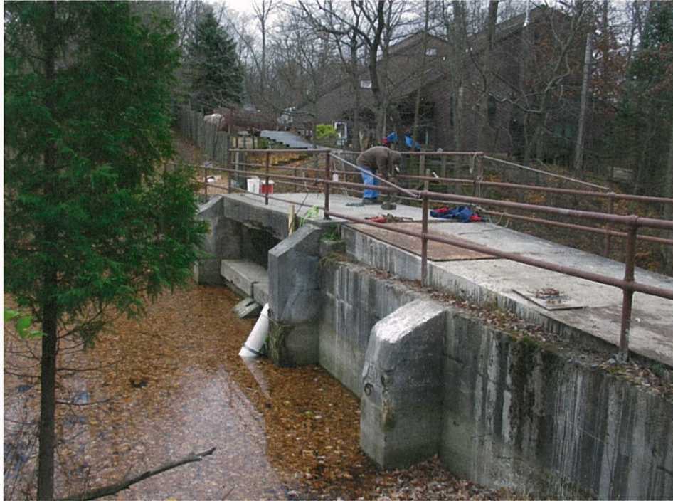
Upstream Face – Looking south-easterly during drawdown
