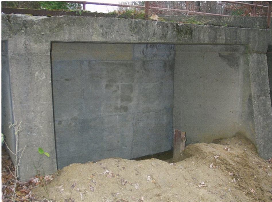
Typical Newly Constructed Wall – Looking at Bay 2
