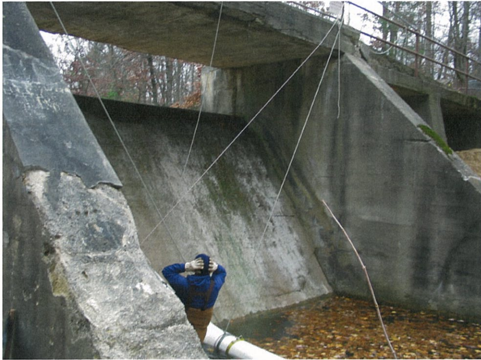
Downstream Spillway – Looking NE prior to spillway patching and sealing
