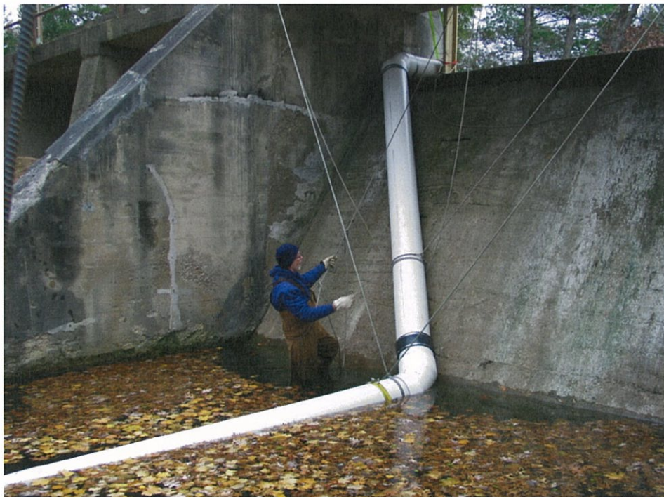
Downstream Spillway – Looking NW prior to spillway patching and removal of temporary siphon tube.
