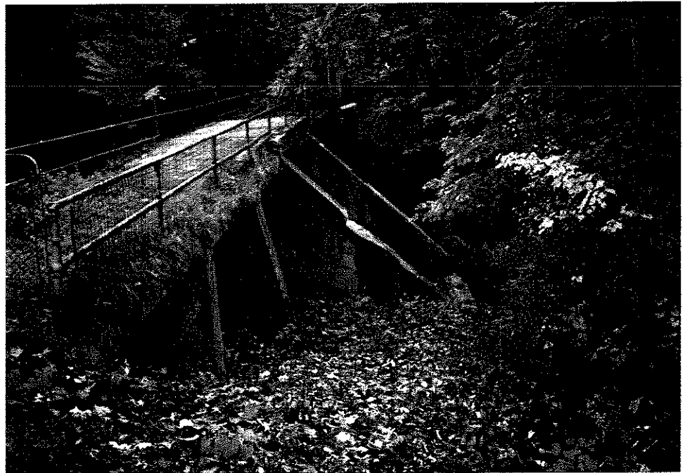
PHOTO #4 DOWNSTREAM FACE OF DAM
