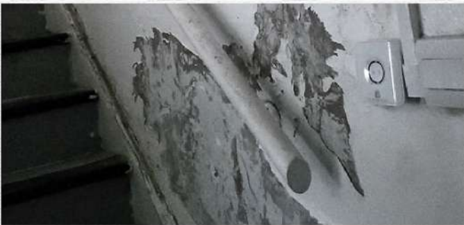
Fig. 4 Plaster crumbling off the walls at Fred Wigg Tower (Simpson, 2022)
