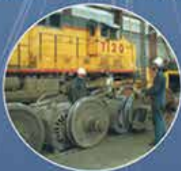
Locomotive Parts & Repair
