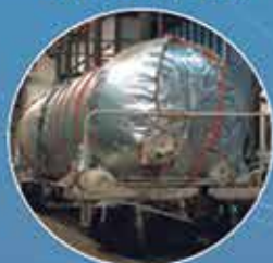
Tank Car Repair
