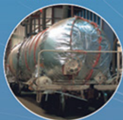
Tank Car Repair
