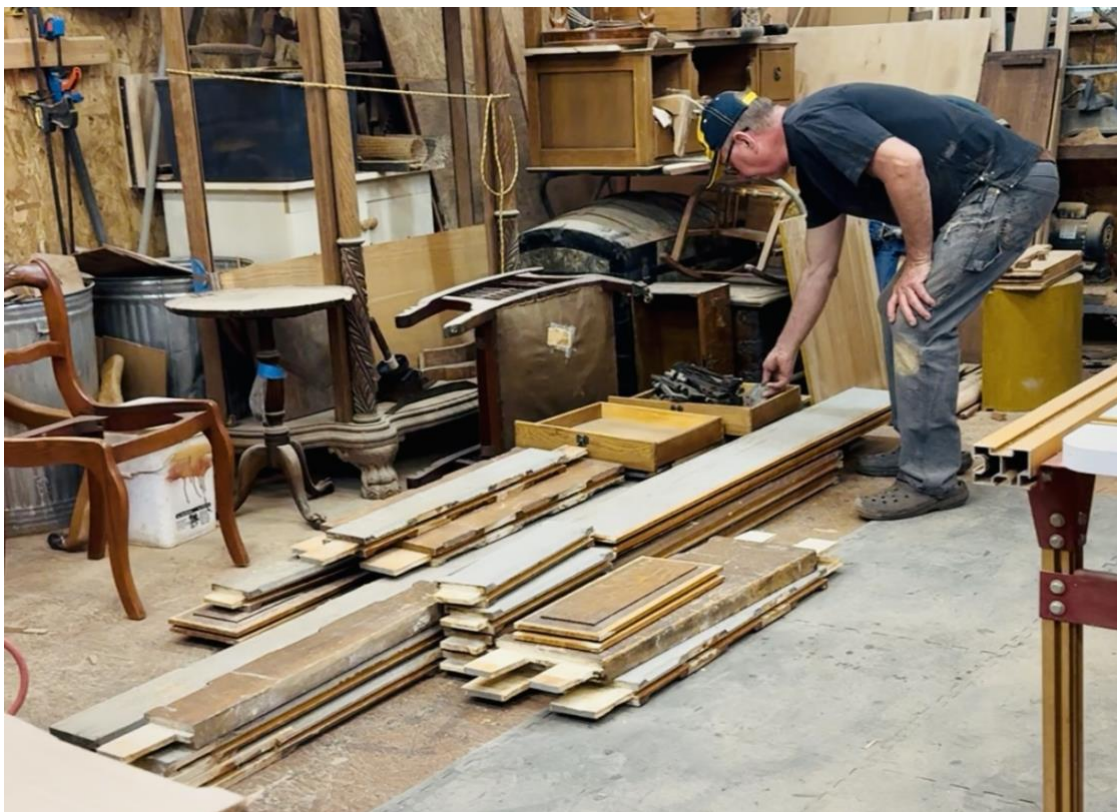
Dismantled interior doors in John's shop
