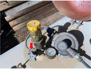
**OPEN valve and light wall heater pilot light.** Often you must bleed air by just holding white push knob for a minute. Keep trying. Turn to I, II or III after pilot lights. Number II is usually more than enough.
