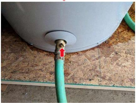
Verify heater block valve OPEN. Turn Left = OPEN.
