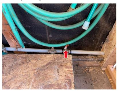
Open hot water heater pressure relief valve. Lift silver handle up. You will Close it once water starts coming out. This step lets you know the hot water heater if full and can be turned on.
