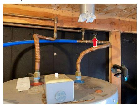
Verity Settling tank drain handle is CLOSED.
