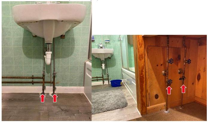
Verify Input Valves are Open (turn to left) on Sink and Tub:
