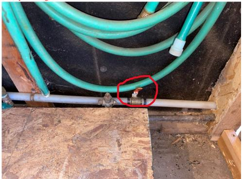
Open heater pressure relief. Lift silver handle up. You will Close it once water starts coming out. This step lets you know the hot water heater if full and can be turned on.
