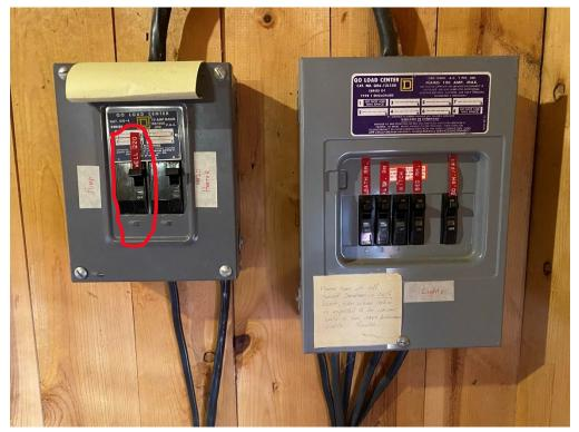
Turn on water heater breaker. (Right breaker in left side breaker box) - Never power the water heater before the tank is full or the elements can burn out.
