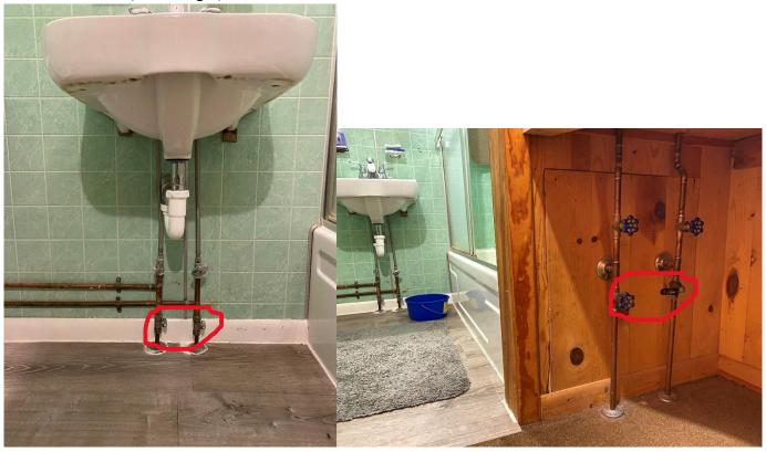
Verify Input Valves are Open (turn to left) on Sink and Tub:
