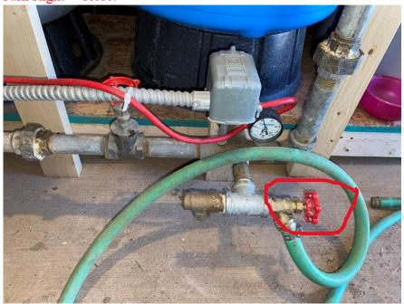
CLOSE heater drain valve. (Requires a flat head screw driver).
