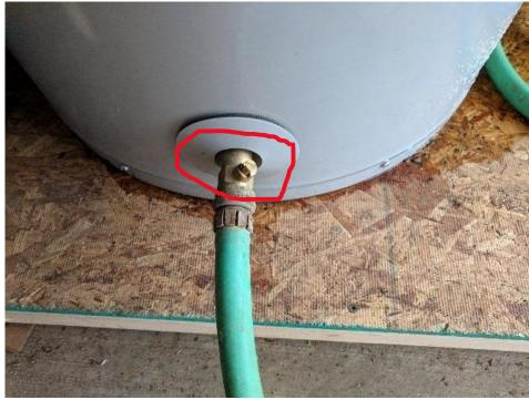
Verify heater block valve OPEN. Turn Left = OPEN.
