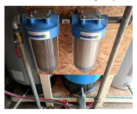
Close washer line drain valves. Turn Right = Close.
