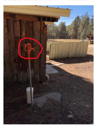
Remove PVC CAP and Turn to On (Open). This opens the valve so water can enter the pump house.
