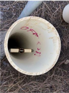
Install water filters. Be sure to lube the black gaskets up! Lube on shelf.
