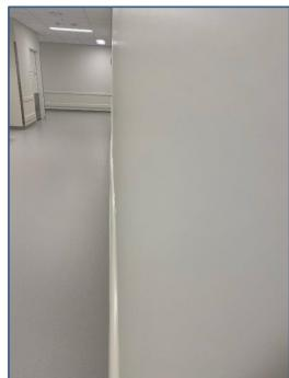
EXPOSED LEAD APRON/ELECTRICAL – SINGLE WALL RADIATION BARRIER WITH UGLY EXPOSED ELECTRICAL CONDUIT AND LEAD APRON EXPOSED WOOD BACKING – AN INFECTIOUS DISEASE NIGHTMARE TO HEALTH FACILITIES.
