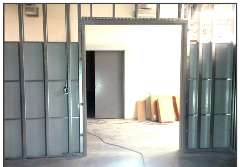
ASRP lead plate installation with entryway shown.
