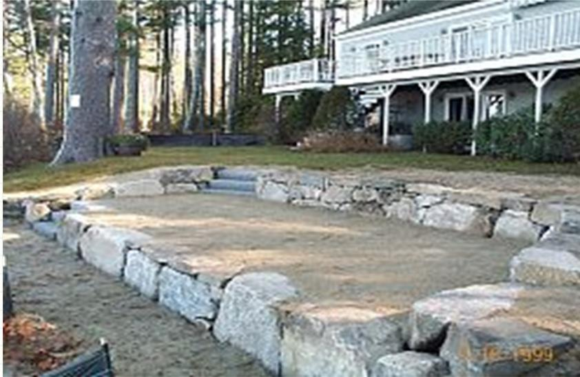
**What is a perched beach?** A perched beach is a beach area that is elevated at least 12 inches above the high watermark. Similar to a garden terrace, there is a retaining wall set along the water's edge with steps allowing easy access to the water; often there is a retaining wall on the uphill side as well to provide a level beach area.
