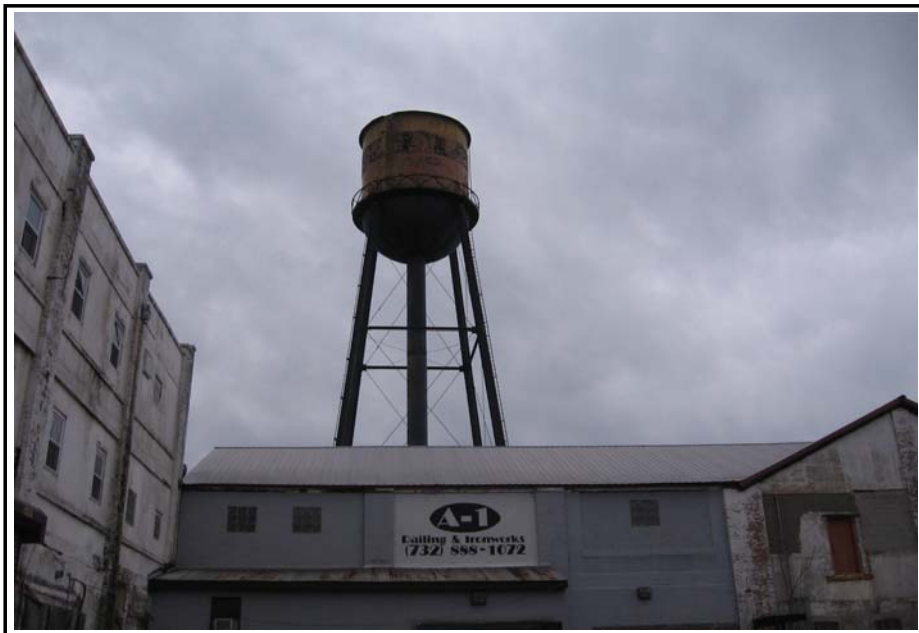
Photo No.: 14 Date: 12/11/2008
