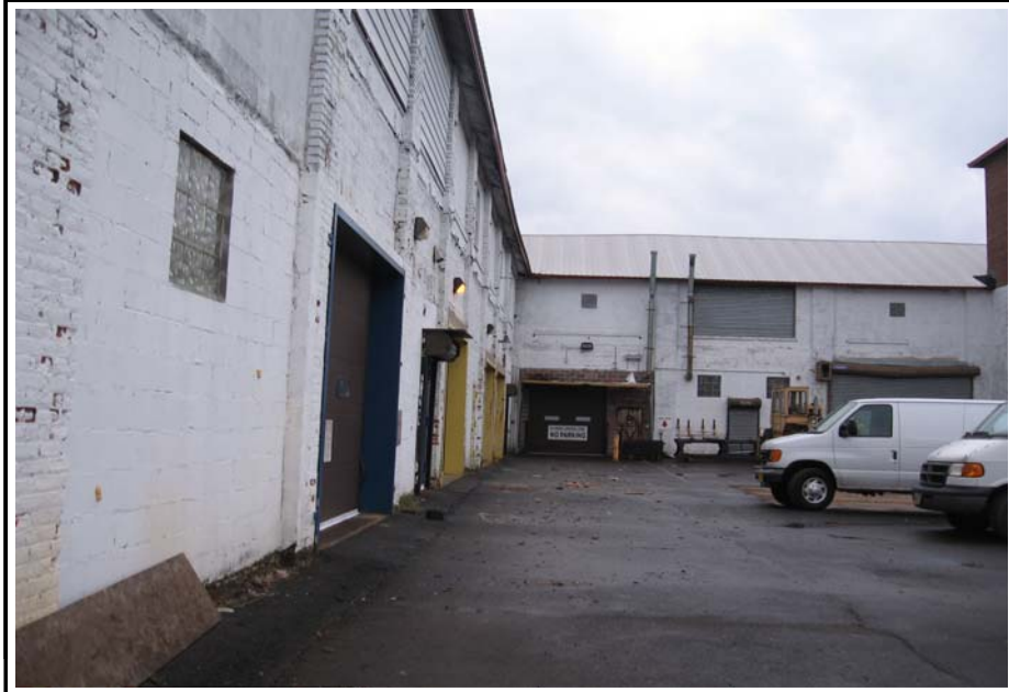
Photo No.: 9 Date: 12/11/2008
