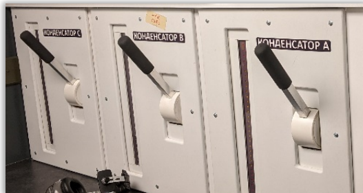
Heater capacitor discharge levers
