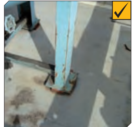
This air receiver is anchored in place by a bolt.
