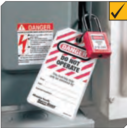
This on/off switch for the air compressor is capable of being locked out.
