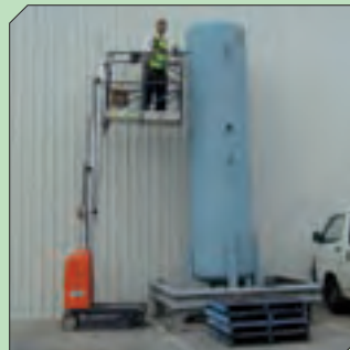
Access platform for servicing the air receiver.
