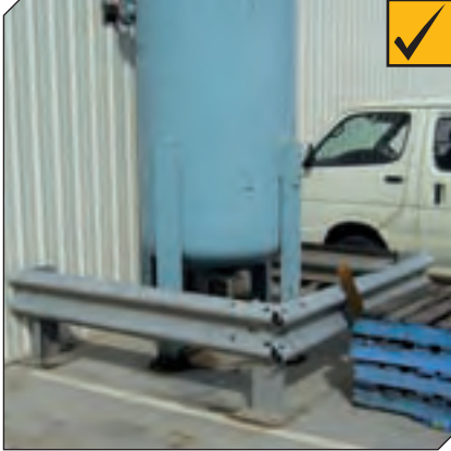
This air receiver is protected from traffic by a properly installed traffic barrier.
