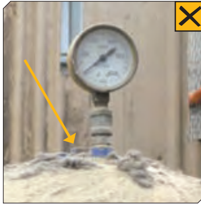
Incorrect: The nozzle for the pressure relief valve has been plugged.
