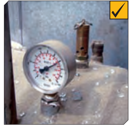
Correct: The pressure relief valve is located behind the gauge.
