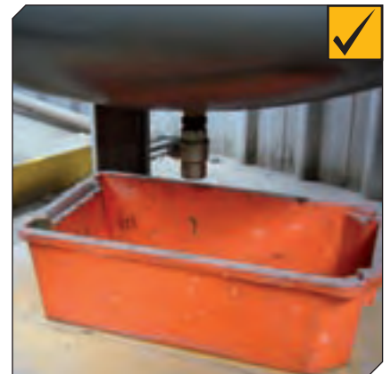
Correct: This blowdown valve discharges into a container so that the oil and water is captured.
