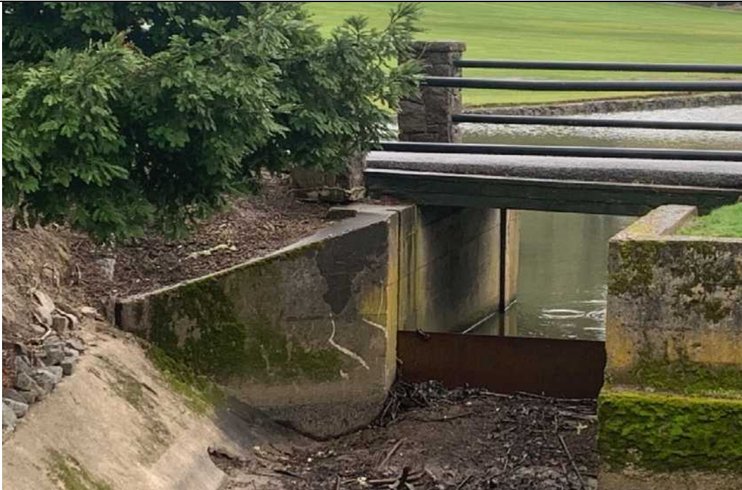
View southeast at water control gate between irrigation pond and Fanno Creek. View of downgradient side of water control gate. Floating debris from Fanno Creek is stopped from entering irrigation pond.
