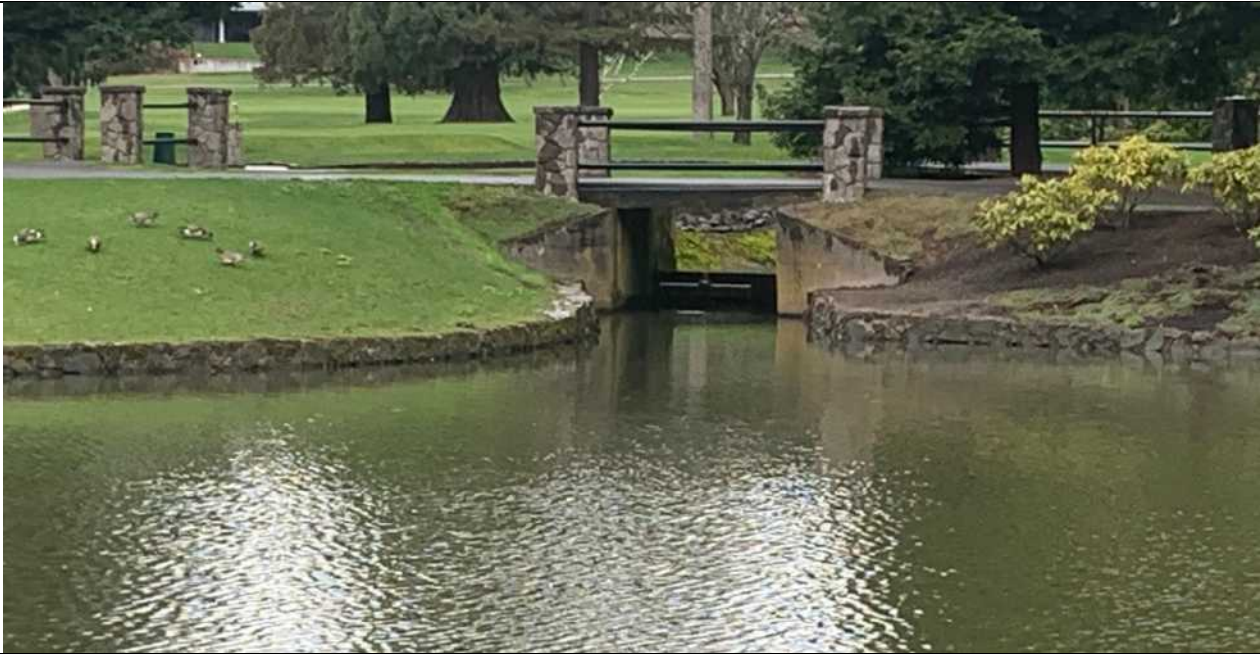
View northwest at water control gate between irrigation pond and Fanno Creek. View of upgradient side of water control gate, which detains water from Woods Creek.
