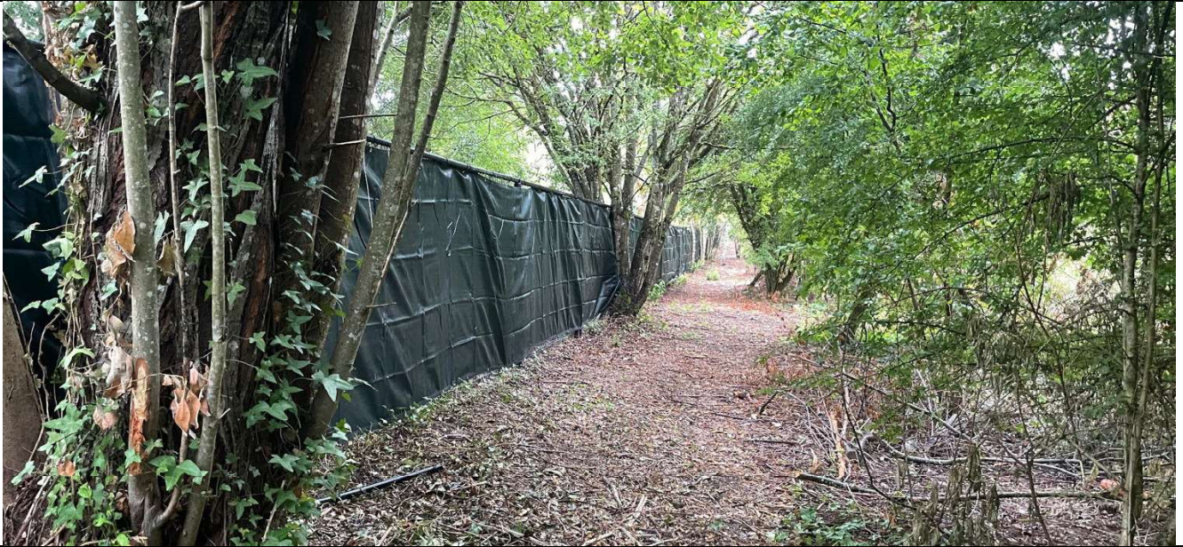
Photo 6. A narrow corridor was cleared when the black fence fabric was installed in July 2024. The clearing avoided larger trees/shrubs (many with multiple stems) and shredded the vegetation into a mulch (no ground disturbance).
