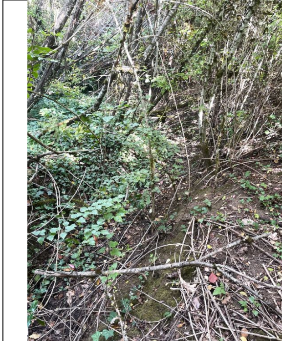
Photo 1 (above): View west at ditch along south side of former railroad berm. This feature amounts 950 sq. ft.
