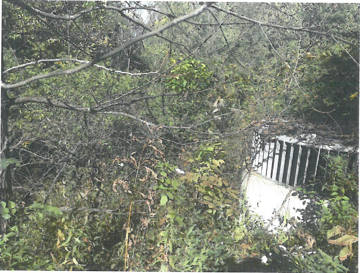
Outlet control structure, facing northwest
