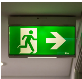
An example of a pictograph emergency light sign.
