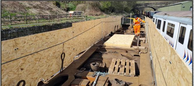
Above: Delivery of wood at the end of March enabled a working party to create a robust safety fence around the chassis
